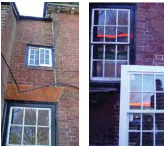
Replicating details and finishes
