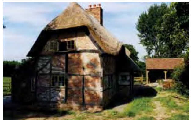
A new timber framed outbuilding.
