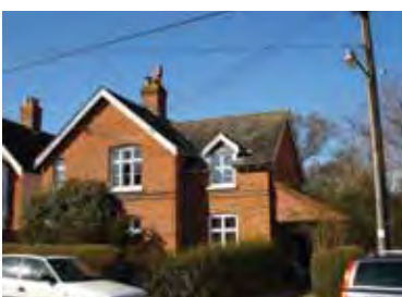
A side extension of diminishing scale, uses matching materials and detail.
