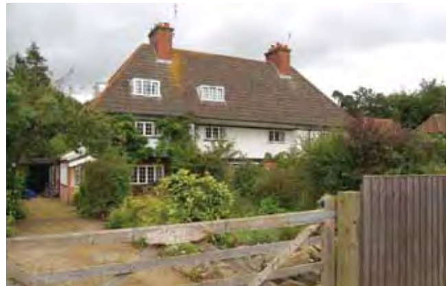
Arts and Crafts style residences and cottages with pantiled roofs at Burley.
