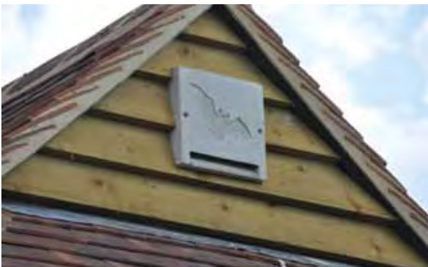
Provision of bat access panel.
