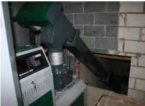
Biomass boiler and housing at Lyndhurst Community Centre.
