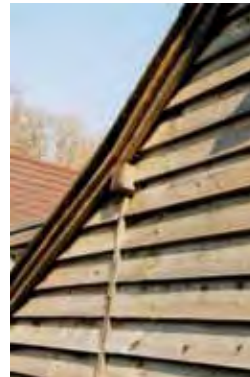
Rustic feather-edged and waney-edged boarding, weathering to a silver-grey. Need to be sizable sections to look rural.
