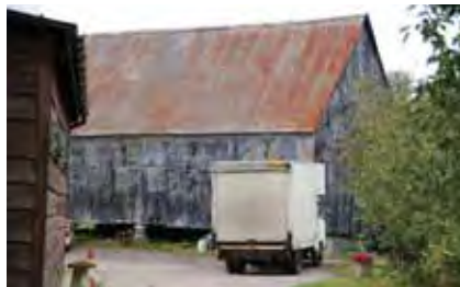
Corrugated iron and other simple profile sheeting can be useful on lightweight structures. Dark toned fibre roofing is also effective.
