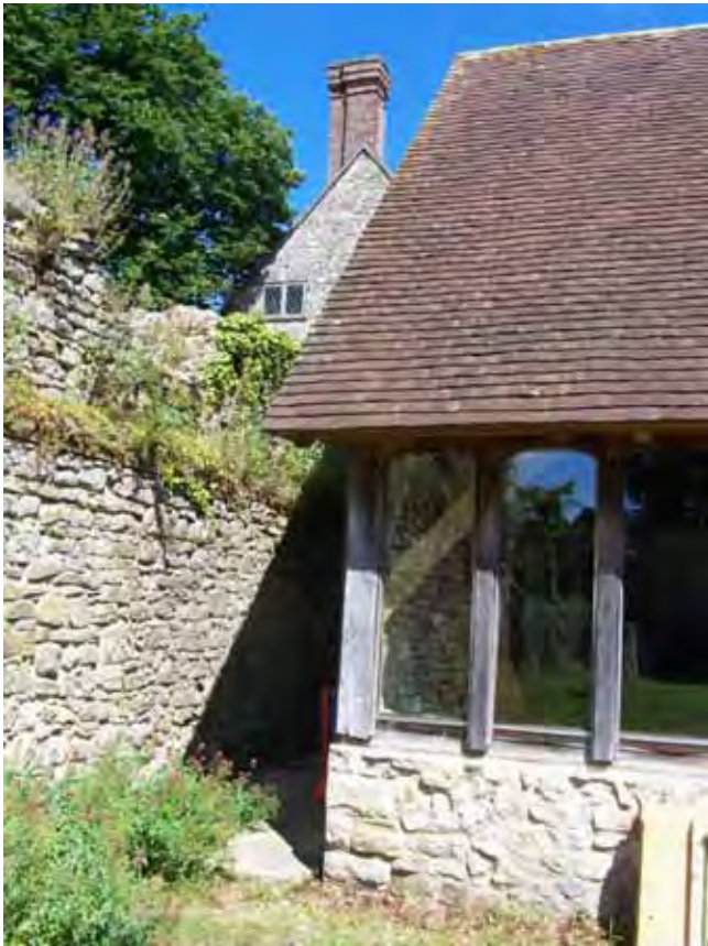
A building responds to adjacent historic buildings and enclosure; using stone, timber, steep roofs and well proportioned window design.
