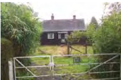
Keeping an original building.
