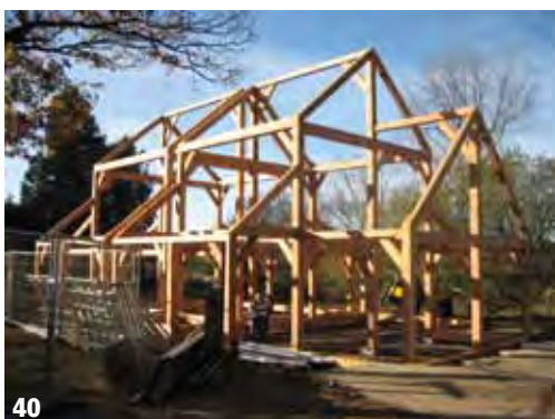
Using construction methods that allow for adaptability and simple dismantling for re-use and recycling.
