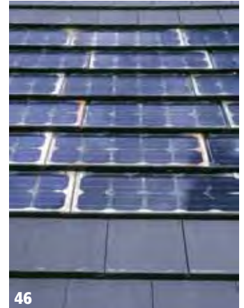
The silvering on some panels and slates can mar overall appearance.
