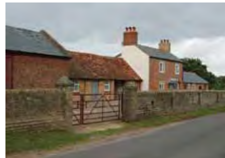
A composition of buildings close to the roadside.
