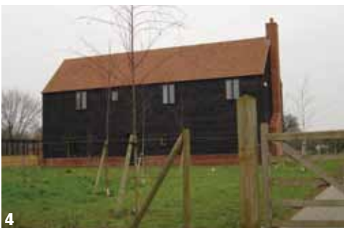
4 A larger scale barn style building, but with space around it to offset its size.
