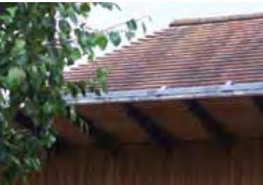
Lead is the traditional material for canopies and architectural dressings, used here in a contemporary design.
