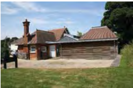
Extending a traditional building with small scale features combined with contemporary elements.
