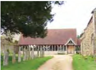
Traditional timber frame, stone and tile complement an adjacent historic building.
