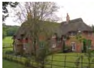
Simple enclosure, estate fencing.
