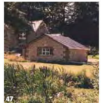
Liquid filled solar slates allow the whole roof to be clad in the same material.
