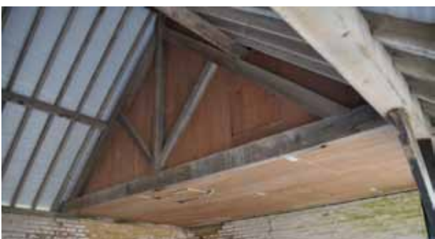
View of bat loft installed inside.
