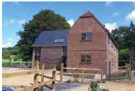
A dwelling looks less bulky by being divided into two or more elements.
