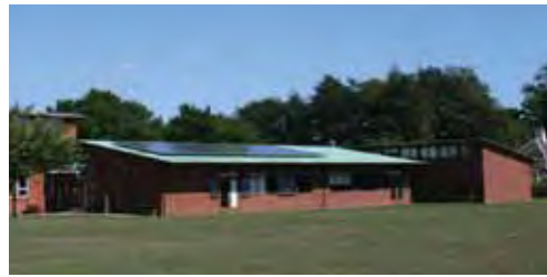
Flush solar panel on a monopitch roof.
